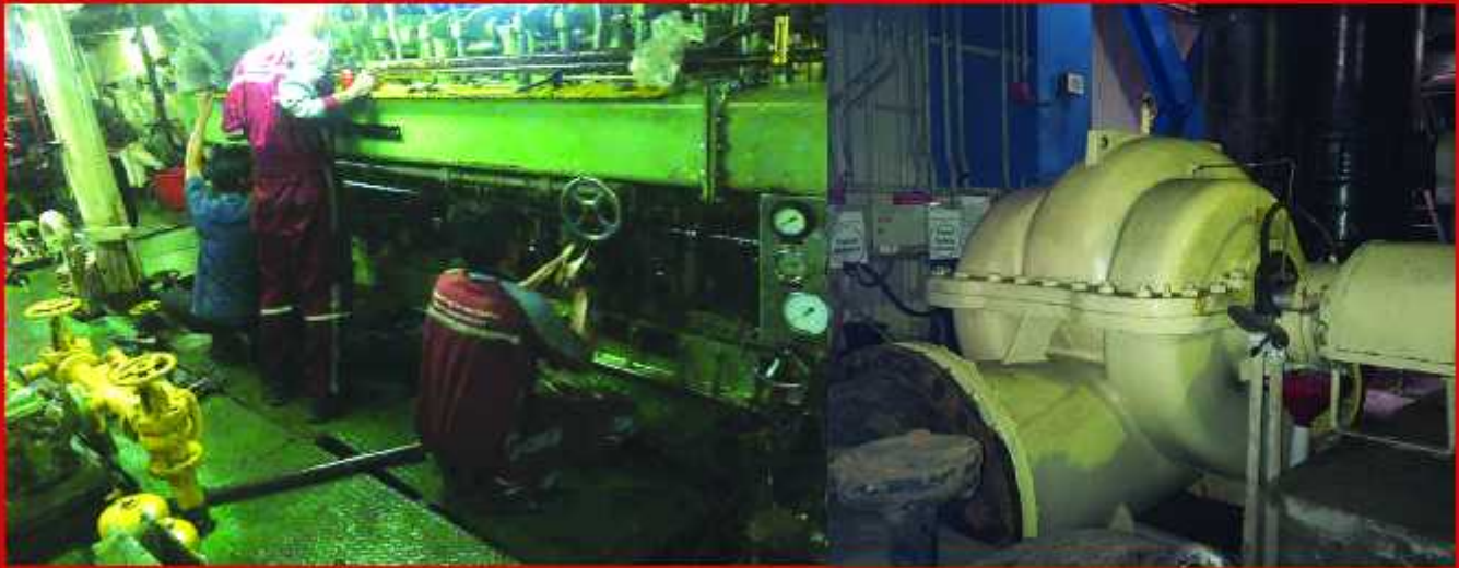
OVERHAUL ENGINE & PUMPS
