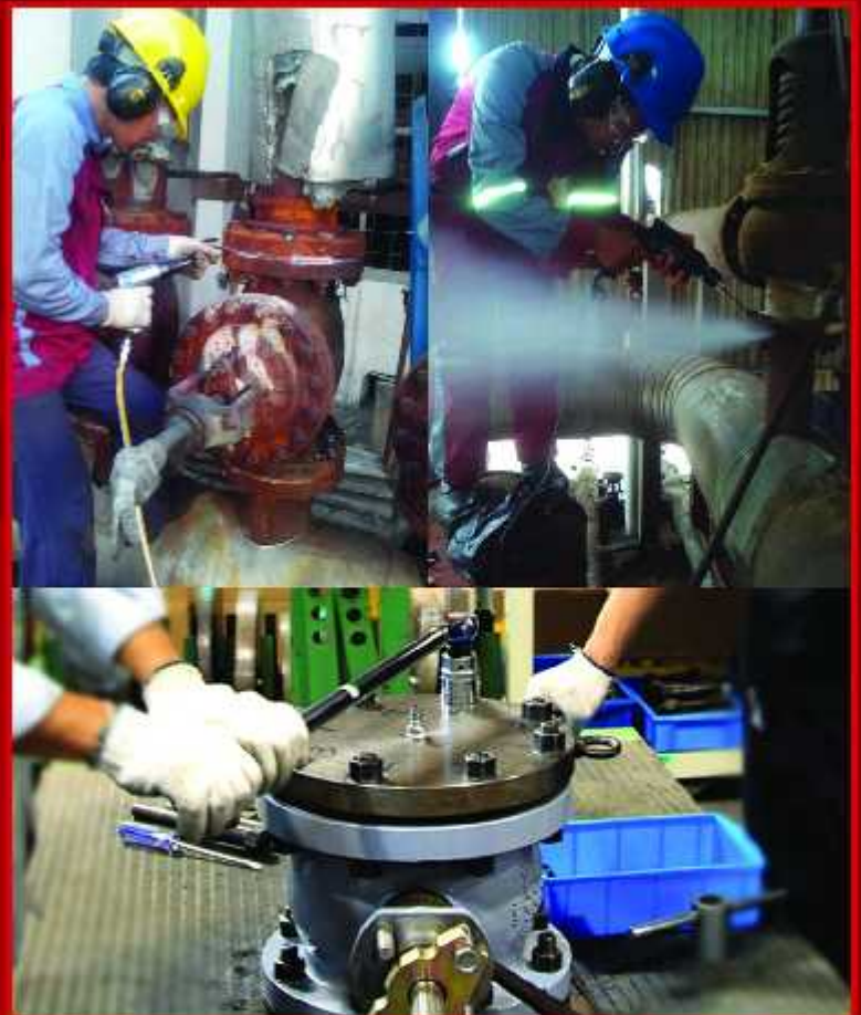
ONLINE LEAK SEALING & VALVES RECONDITION
