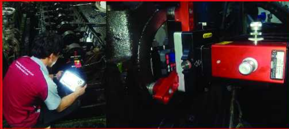
IN SITU LASER ALIGNMENT
